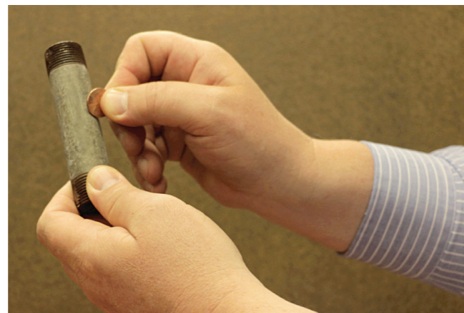
Galvanized Steel Pipe The scraped area remains dull and gray.
